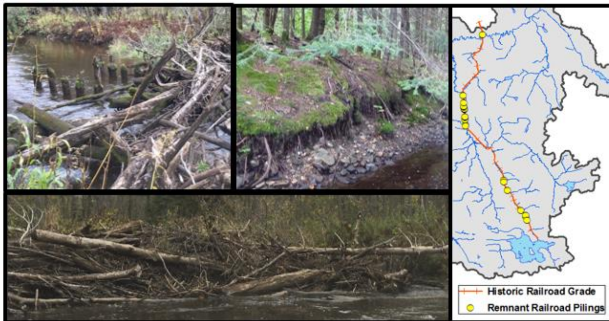
Figure 15. Map (Right) identifying locations where the old railroad historically crossed the Ash and Blackduck Rivers including one location on the Ash River and 18 on the Blackduck River. Pilings remain in the stream at many of these historic crossings causing debris pile-ups (top left and bottom). Bank erosion was identified in the Blackduck River in areas where the old railroad runs parallel with the Blackduck River (Top center).
