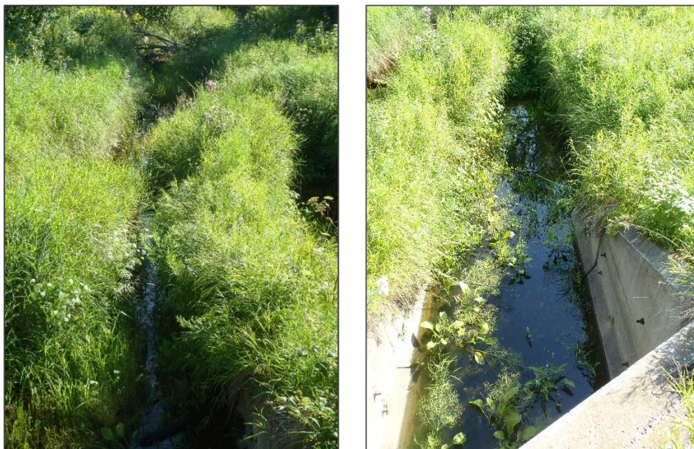
Photo 8. Perry Creek at Buckeye Road, August 3, 2016, looking downstream. Of the paired culverts at this crossing, the left photo is the culvert that carries more of the low flow. The right photo (and right culvert) is a bit out of the channel/thalweg and has accumulated some sediment below the outfall. Emergent aquatic vegetation is growing inside the culvert (very rarely observed), suggesting frequent low flow volumes or stagnant conditions (as it was here).
