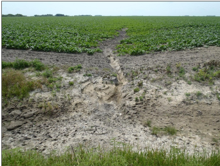
Photo 8. Surface erosion from an unvegetated field swale along State Highway 75. A significant delta of soil has been deposited in the ditch, where it can move downstream farther. There were several of these from this
