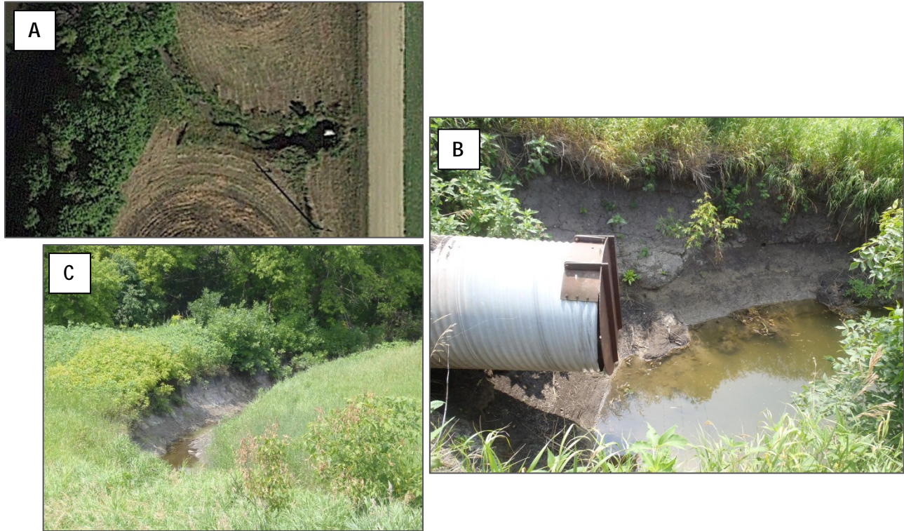
Photo set 5. A large road culvert on Township 140 was found that is installed such that it is creating a very large, eroded scour pool, and the channel below continues with raw, eroding banks. A) Aerial view – the trees on the left are growing on the bank of the Rabbit River, B) Ground photo of the scour pool. The culvert bottom is about six feet above the water surface, and erosion has occurred back almost to the road bed, C) The raw channel below the culvert.
