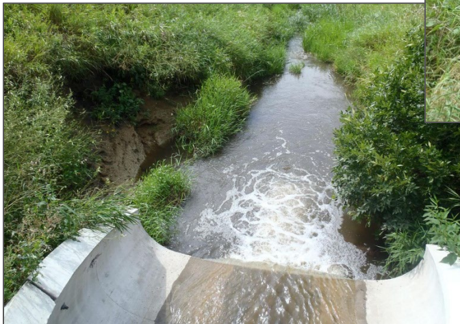
Photo 25. This new culvert on CR-66 is installed with the downstream end perched above the ditch's water level, making it impassable for fish needing to go upstream.
