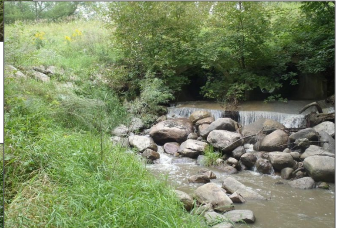
Photo 24. The culvert outlet at the Township Road 18 crossing is elevated by about two feet above the stream water level.
