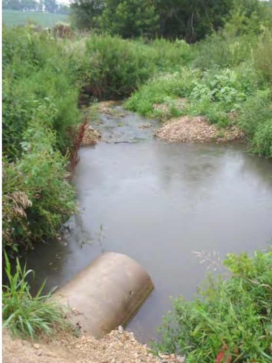
Figure 136. Upstream of biological Station 08LM087; at road crossing (potential culvert impacts on stability)
