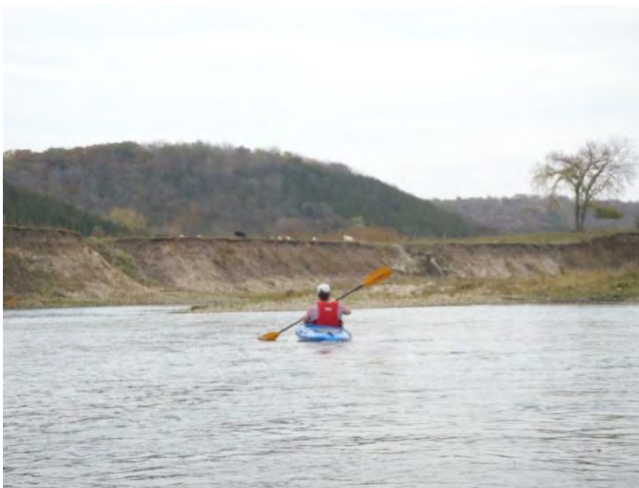
Figure 148. Kayak reconnaissance photograph, October 10, 11, showing incised channel and instability accelerated by land use and lack of vegetation, near Station 08LM070.
