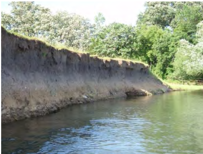
Figure 114. Bank erosion at 08LM005.
