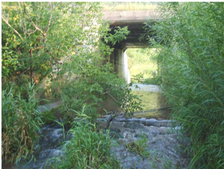
Figure 128. The upstream end of biological monitoring Station 08LM103, looking upstream at culvert on John Deere Road
