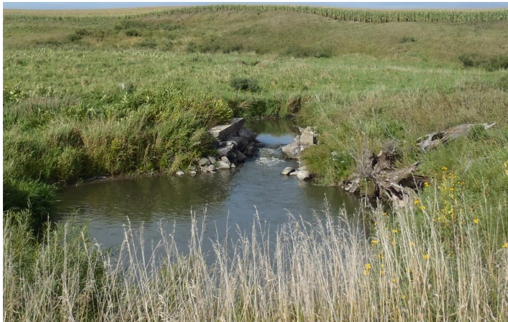
Figure 51. Fish barrier at station 15MN039 (9/16/14)
