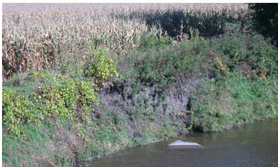
Figure 89. Eroding bank at station 15MN079 (10/30/17)
