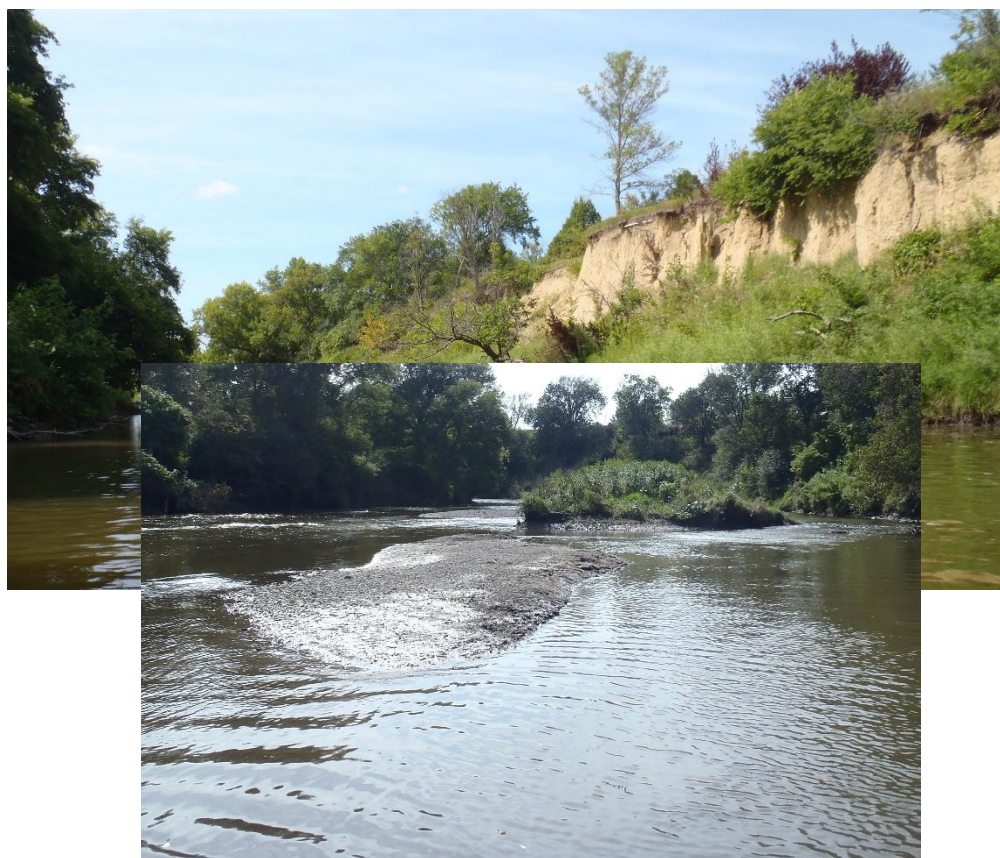
Figure 81. Severe bank erosion at site 10EM003 on 8/4/15 (top) and a sandbar from excess sedimentation at site 15MN082 on 9/15/15 (bottom)
