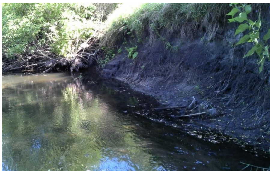
Figure 15. Erosion at site 15MN072 (8/12/15)
