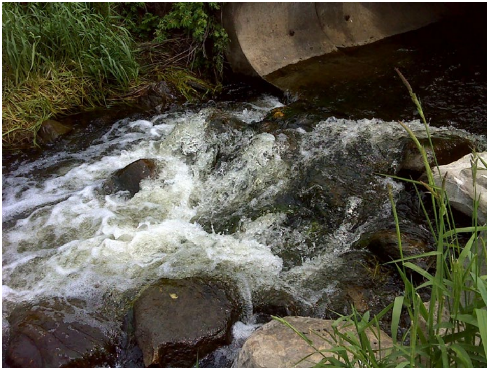
Figure 41. Culvert at station 12UM025 (June 11, 2014)
