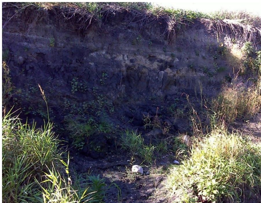
Figure 114. Erosion at station 12UM006 (October 9, 2013)
