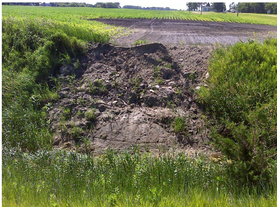
Figure 98. Field erosion on tributary to 12UM067 (July 8, 2014)
