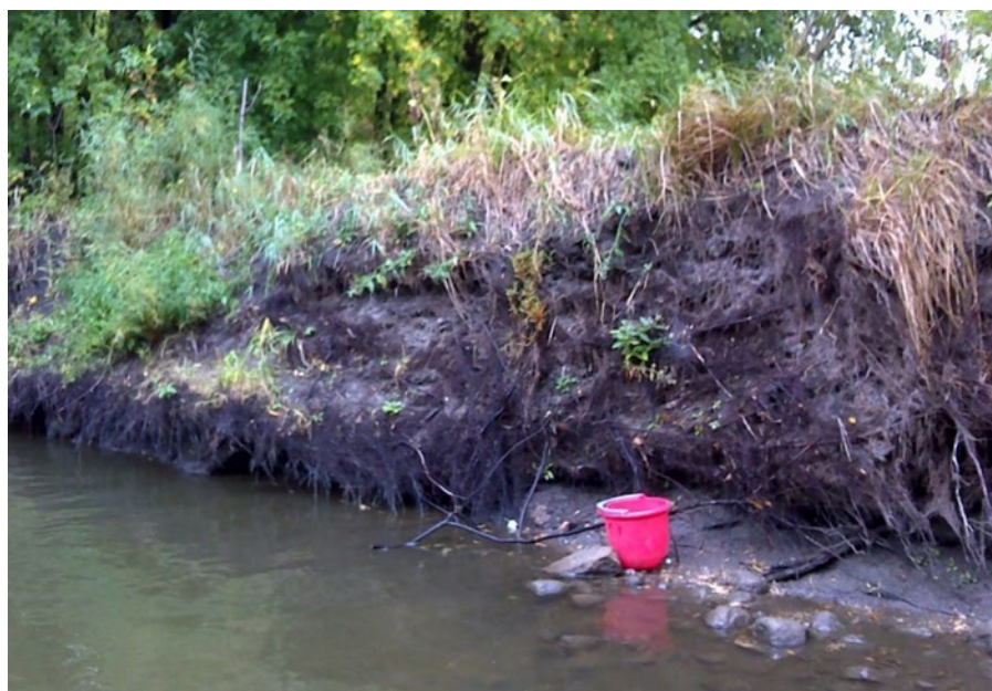
Figure 68. Eroding bank at station 14UM001 (October 3, 2013)
