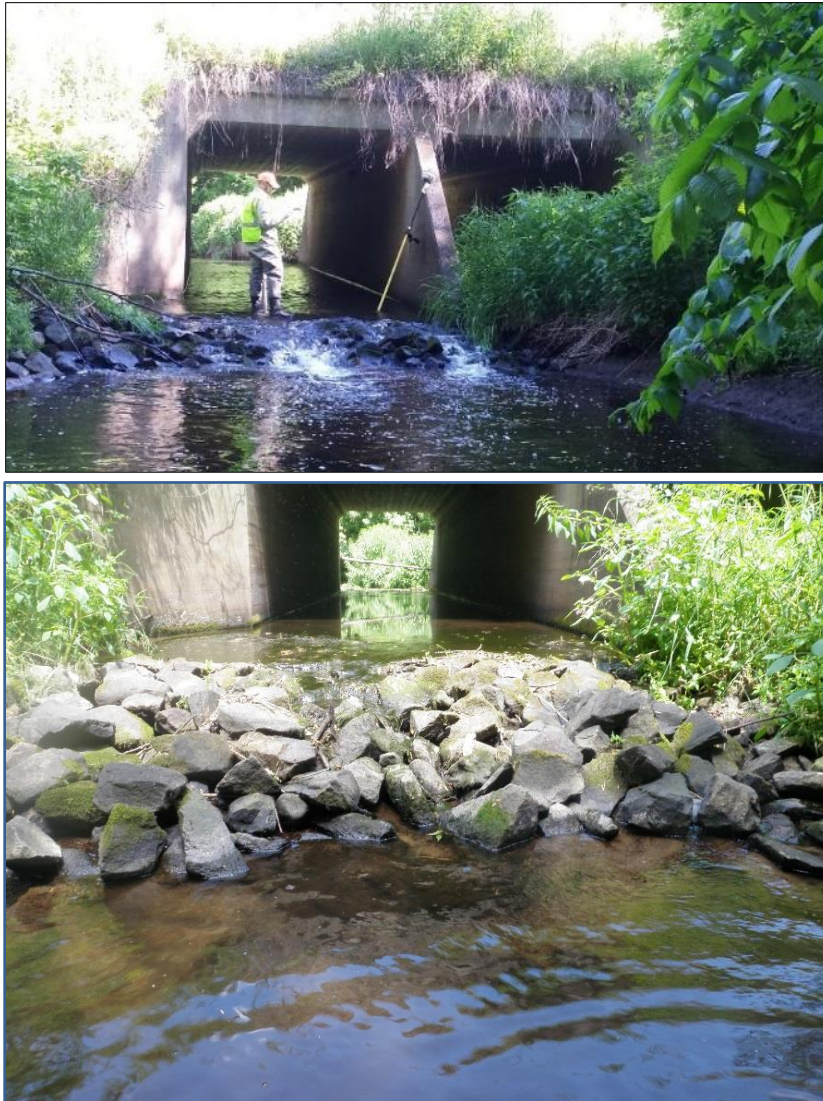
Figure 94. Pictures of the Zuleger Creek crossing with Benton County Road 12, illustrating the barrier to fish passage.
