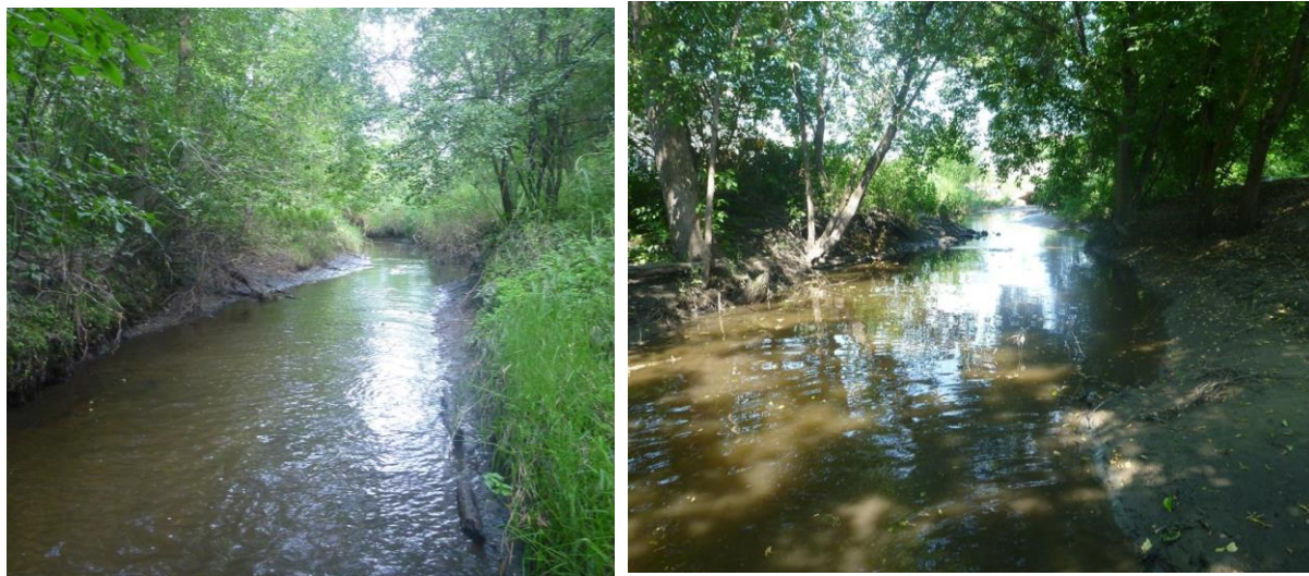
Figure 71. Pictures of Stearns CD13 (near Sartell, Minnesota) taken on 8/3/2016, courtesy of MN DNR. The ditch shows signs of channel instability, such as bank erosion, widening, and channel incision.
