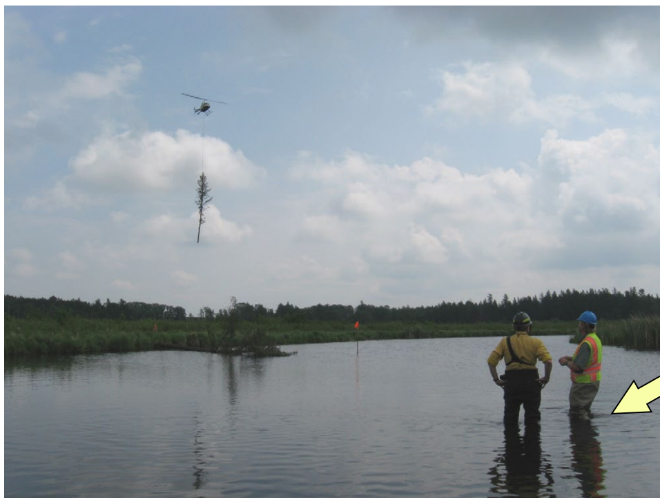
Photo 13. MDNR deemed that parts of the adjacent Straight River needed habitat enhancement due to the absence of structural habitat/cover and channel forming materials. Trees were imported and carefully placed to enhance the naturally bland, homogeneous channel morphology. MDNR Photo
