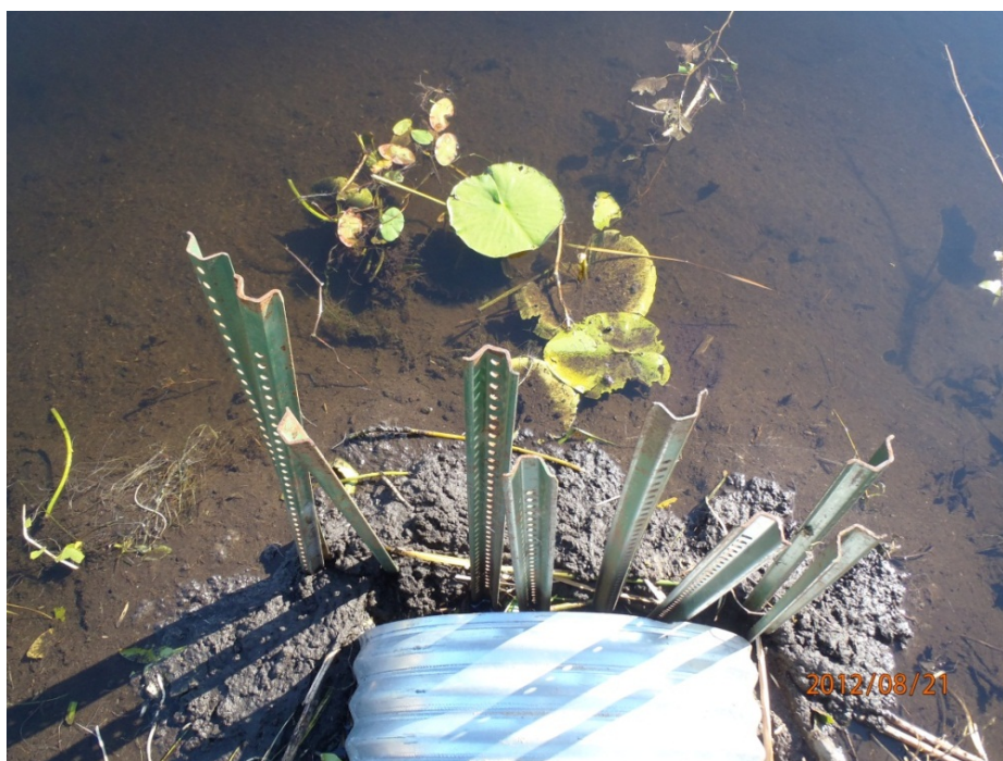
Photo 6. Outlet of Tripp Lake wetland, blocked by a mud beaver dam. There was evidence here of repeated attempts to maintain open flow in this culvert (debris pile, stakes over culvert opening).
