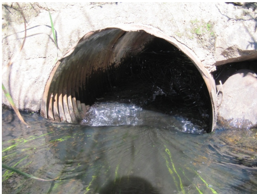
Photo 5. Upstream entrance to the Aspen Lane culvert. The culvert elevation is not correct, and it is also undersized, causing the flow to be quite swift.
