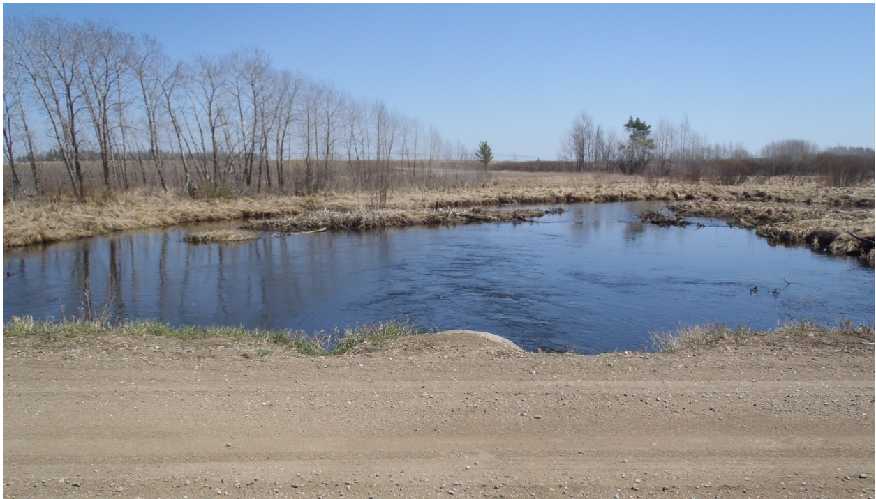
Photo 20. Culvert at 520 th Ave. Strong velocity was observed coming from the culvert, which is undersized, and this large scour pool is the result of these more-erosive flows.
