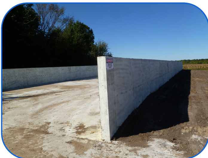
Completed Manure Stacking Slab
