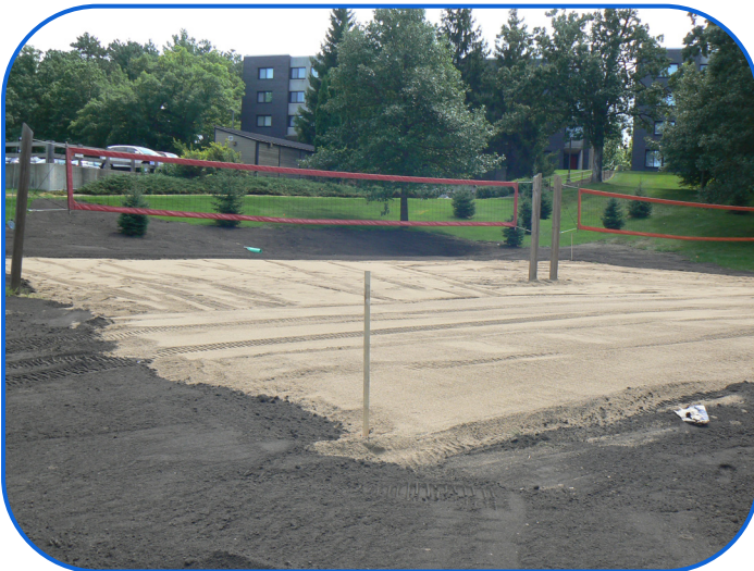
Volleyball Court Amended to a Infiltration Basin
