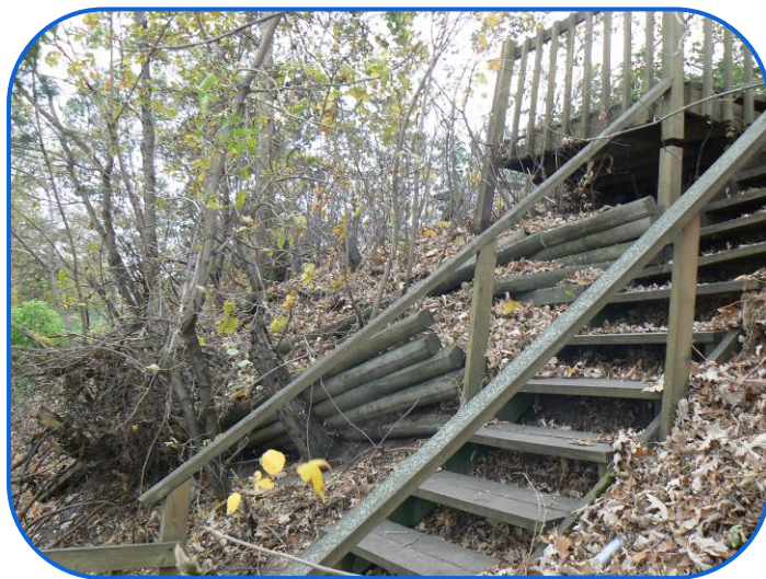
Failing Retaining Wall System
