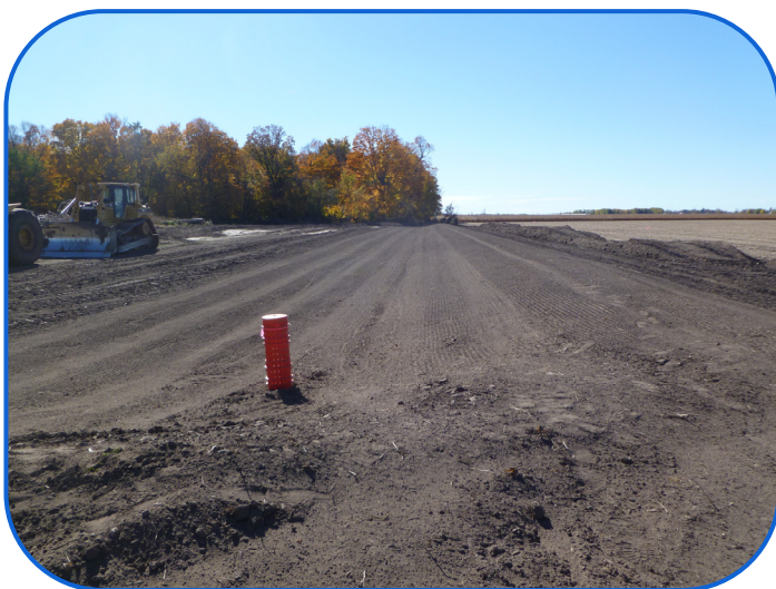
Water and Sediment Basin with Control Inlet
