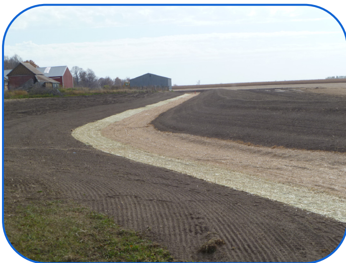
Grassed Waterway Shaped, Seeded and Erosion Blanket
