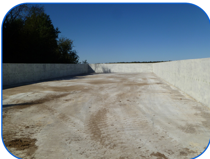
Completed Manure Stacking Slab
