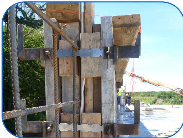
Forming of Concrete Stacking Slab Walls
