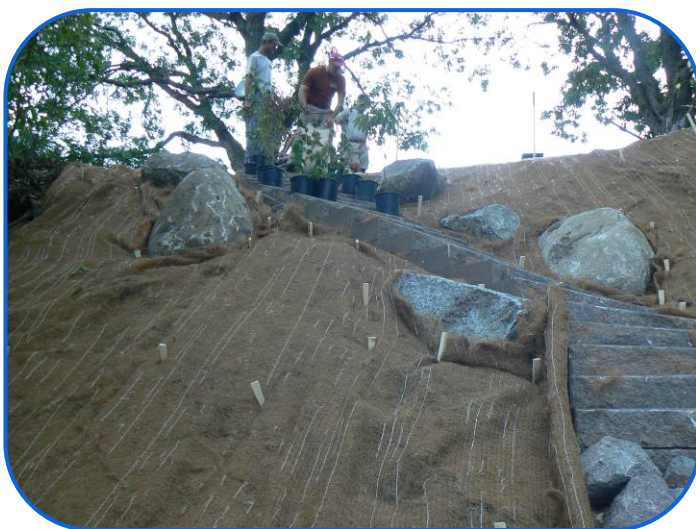
Erosion Blanket & Plant Installation
