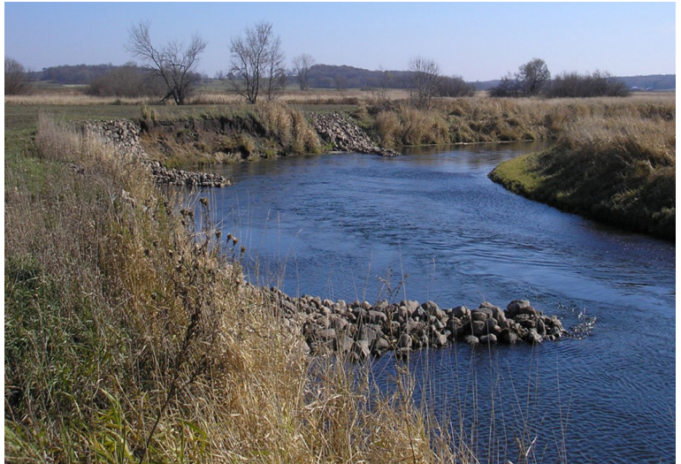
Long Prairie River, showing eroded bank and completed streambarbs. Photo from Shannon Wettstein
