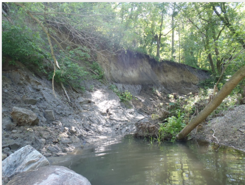
Figure 24. Images of severe bank failure present within station 10RD019 located on County Ditch # 52
