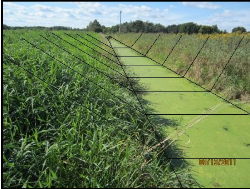
Figure 52. Geometry of constructed agricultural ditches across CCWD.
