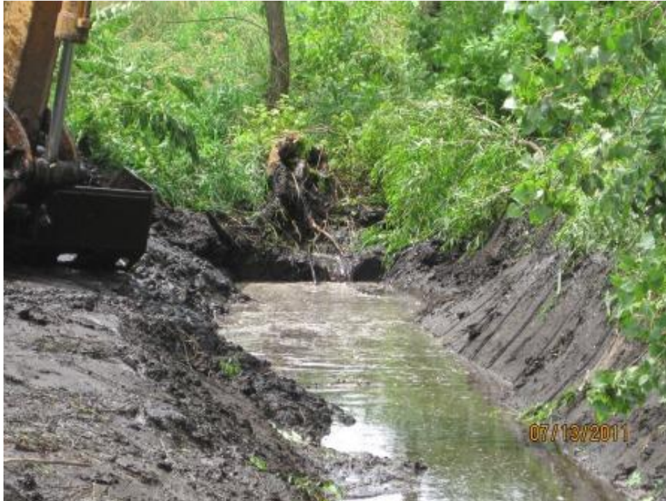
Figure 37. Channel in the process of being dredged.
