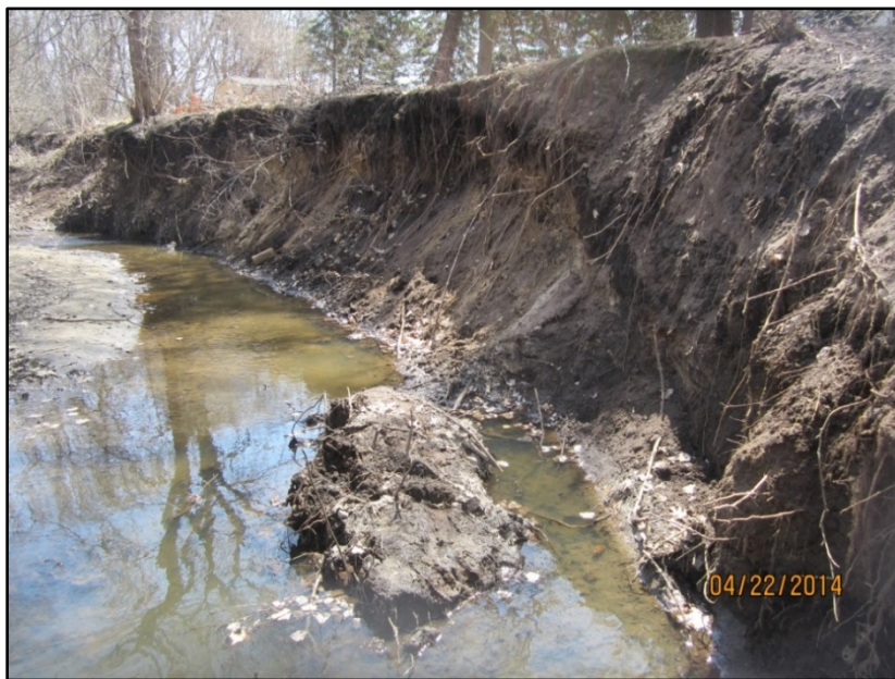
Figure 11. Streambank erosion in Coon Creek Subwatershed.
