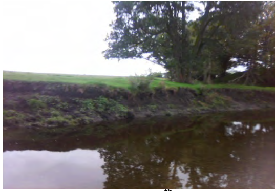
Stony Creek upstream of 325 th Ave
