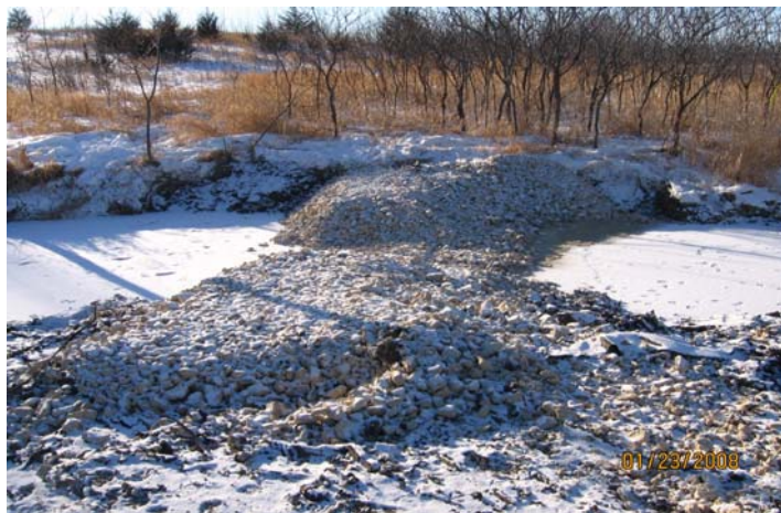
A diversion berm was constructed in December 2007 to divert stream flow into Segner Pond, a sedimentation basin on the Cedar Lake inlet.
