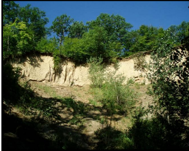
Figure 4.28 Large slope failure with wet soils on lower area and dense sandy clay soils on upper bank (Site 14)
