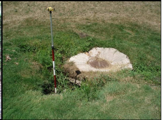
Figure 4.9 Pipe inlet in poor condition from east end of golf course parking lot (Site 4)
