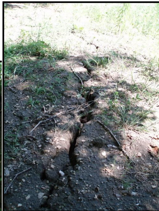
Figure 4.15 Crack foretelling impending slope failure (Site 7)
