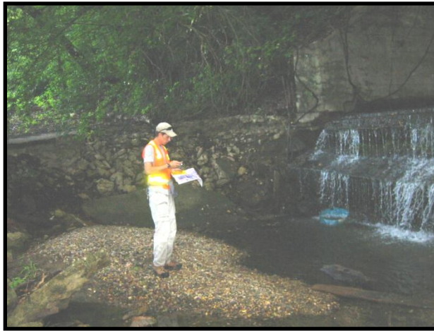
Figure 4.2 Large drop and undermining at downstream end of regional trail culvert (Site 1)
