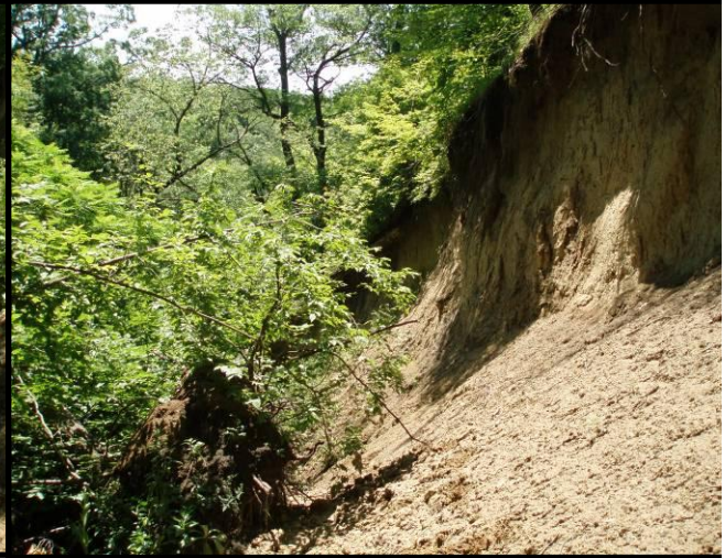
Figure 4.21 Failed sidewall (Site 10)
