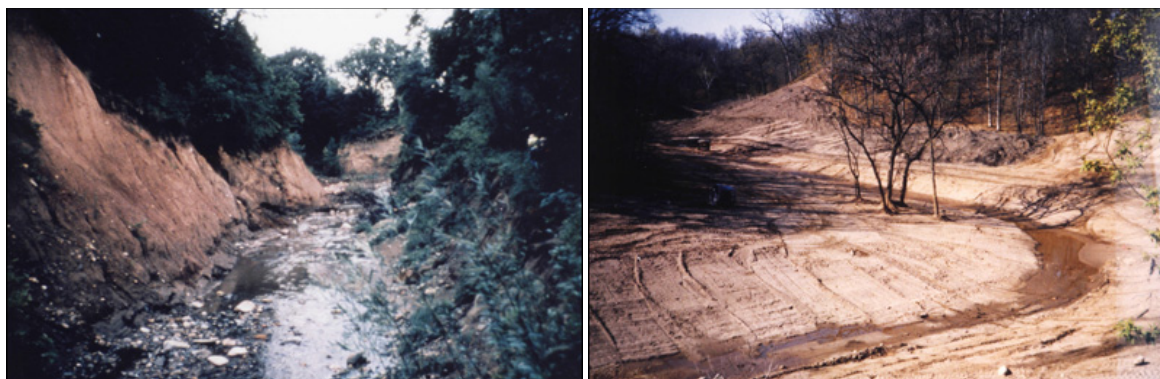
Figure 4.20 Severe pre-Battle Creek Project bank erosion (left) and regrading efforts during construction (right).
