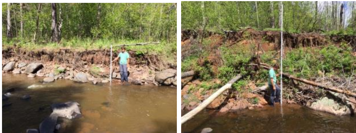
Figure 10. Category 3 Erosion Rates Observed in Reaches AM-2 and EB-2 (0.3 to 0.5 ft/yr).
