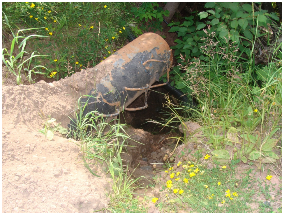
Figure 21. Perched culvert.
