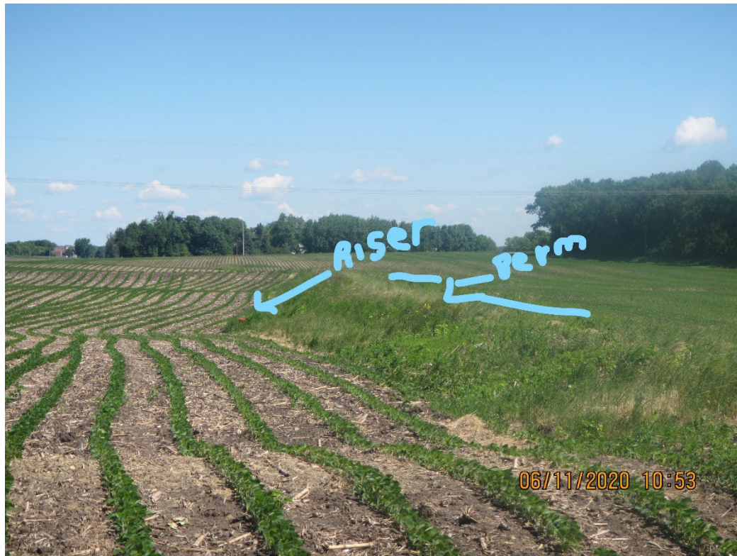
Figure 20. WASCOBs are a common best management practice in the Twelve Mile Creek Watershed. In this photo, the grassed berm on the right holds back water until it becomes high enough to drain through the orange riser on the left, providing storage that helps water quality.
