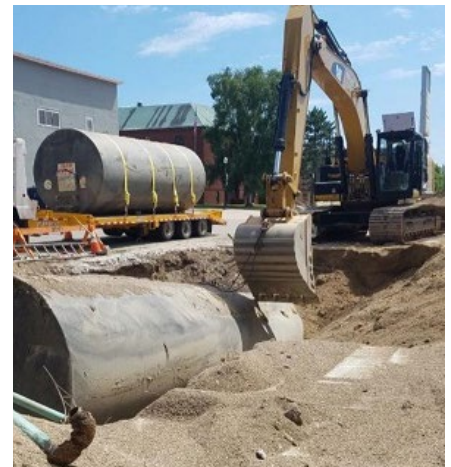
An abandoned fuel storage tank is removed to protect the public water supply in Bovey, MN.
