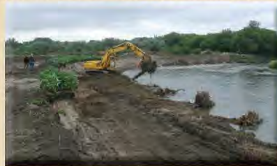
Installation of root wads using an excavator to drive tree trunks into the bankfull bench (looking upstream).
