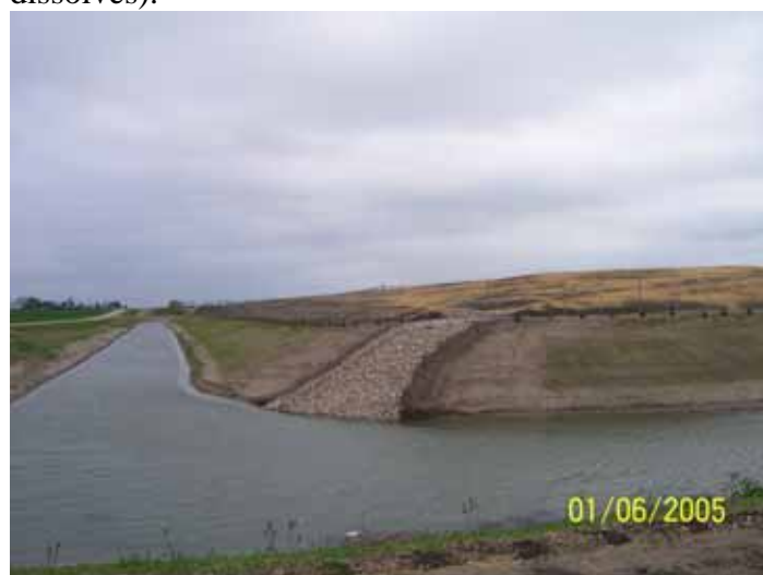
Riprap drainageway off final cover into perimeter sedimentation pond at Clay County Landfill.
