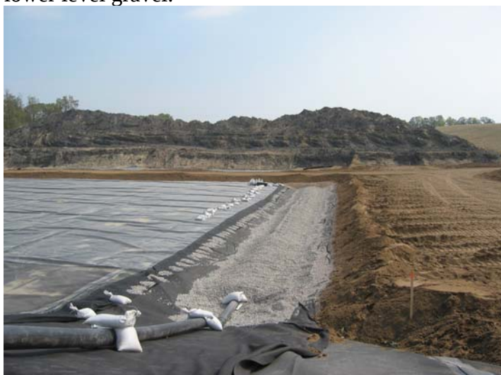
Gravel placement in leachate collection trench at the NE Otter Tail Landfill.
