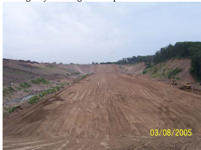
Sand drainage layer in completed cell at Elk River Landfill.
