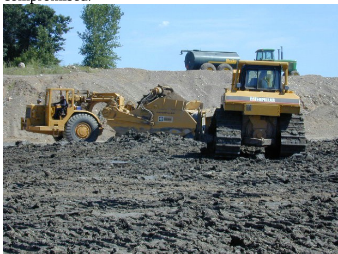
Clay liner construction at the Morrison County Landfill.
