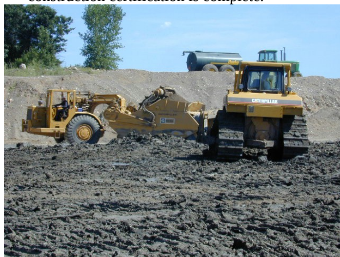
Liner construction at the Morrison County Landfill.
