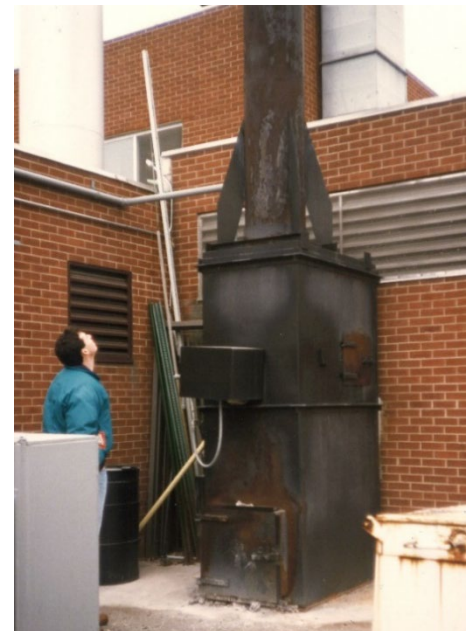
Figure 1: This photo from 1990 shows a medical waste incinerator, and similar ones were used at grocery stores. Practices like this are now banned in Minnesota to reduce exposures to the harmful air pollutants that were released.
